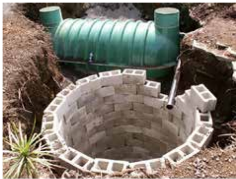
Orenco 1,500-gallon tank and block-lined seepage pit.
