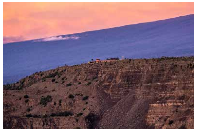
The former Jaggar Museum, and two buildings operated by the U.S. Geological Survey Hawaiian Volcano Observatory, the Okamura Building and the Geochemistry Annex, are slated for removal starting Monday, April 8. Restrooms at Uēkahuna will temporarily close for the duration of the deconstruction project. Portable lua (restrooms) will be available. Ranger programs will continue.
