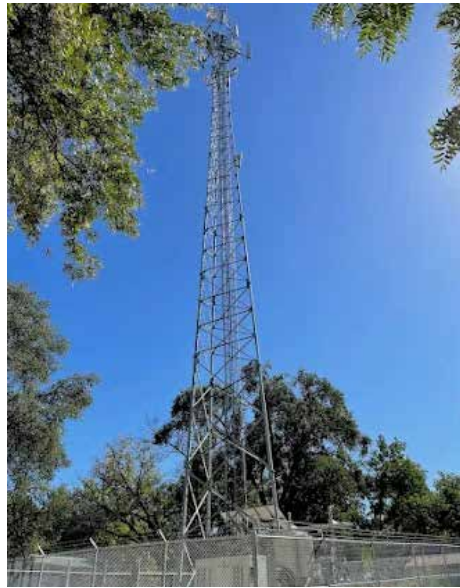
Example of 150 ft. tall cell tower, this one in Round Valley, CA. Photo from Mendocino Voice phone tower on the proposed one-acre site:
