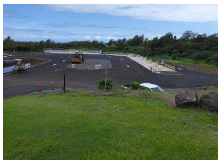
The new Wai'ōhinu Recycling & Transfer station. Photo by Ann Bosted
