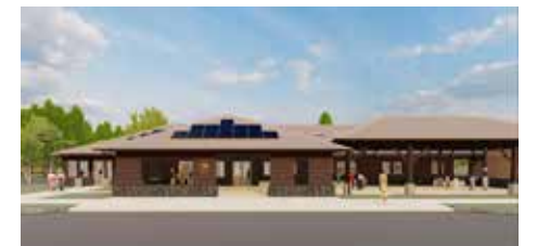
Proposed new visitor center for Hawai'i Volcanoes National Park. Image from National Park Service
