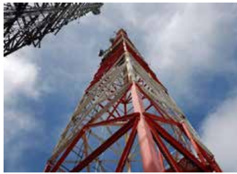
The tower at Kulani Cone, with new transmitters sending two Hawai'i Public Radio station streams, HPR-1 and HPR-2, further into Volcano and Ka'ū, following acquisition of the KAHU community radio license in Pāhala. Photo from HPR
